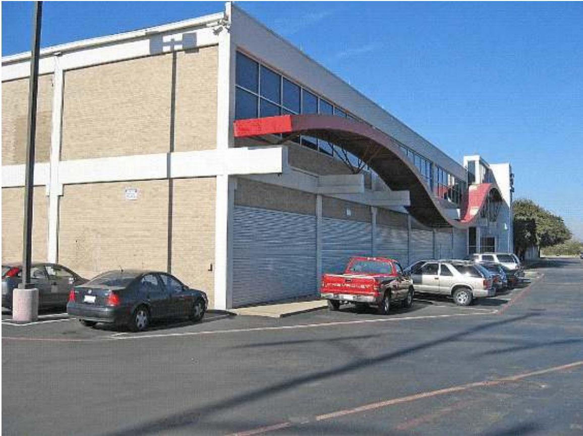
Data Center, Dallas, Texas
